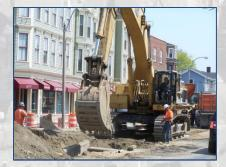
Sewer separation Added capacity & off-line storage: Union Sq. to CMI via Somerville Ave.
