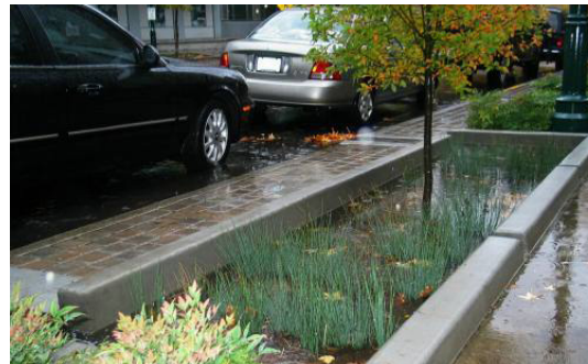
Figure 4.1-4: Rain gardens like this one can alleviate drainage issues
