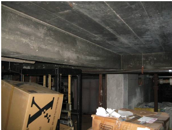
Concrete structure at basement ceiling- the first floor can support heavy assembly loads.
