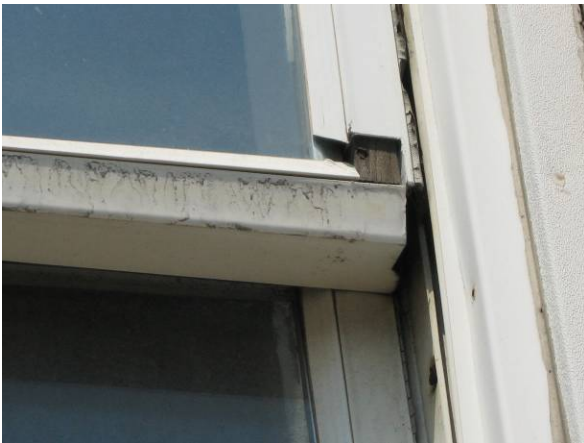
A typical window – all need replacement
