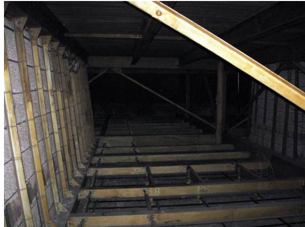
Truss space adds approximately 10' to 1 st flr. height
