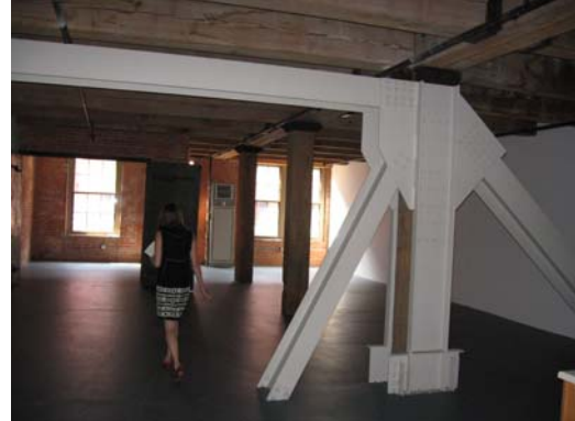
Trusses were retrofitted into the building to carry the residential floors above.
