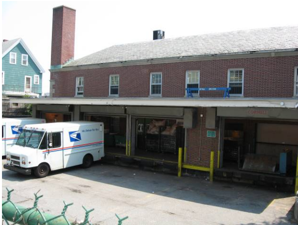
Loading area with truck level dock and canopy
