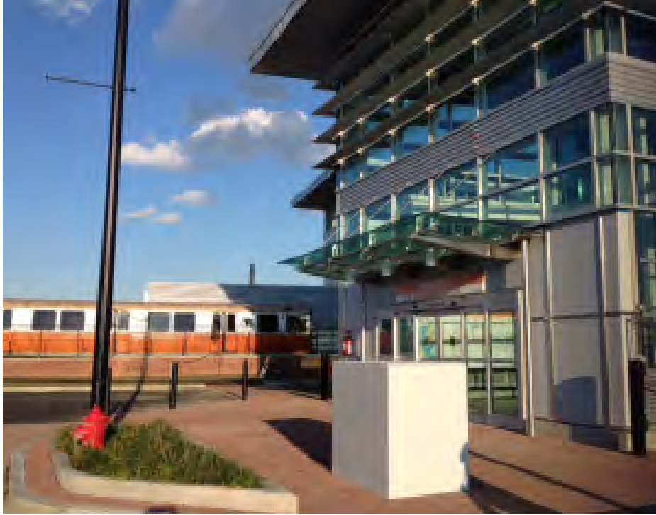
The new Assembly Square Orange Line station, funded with a combination of federal, state and private funding, was the first new MBTA station since 1987.
