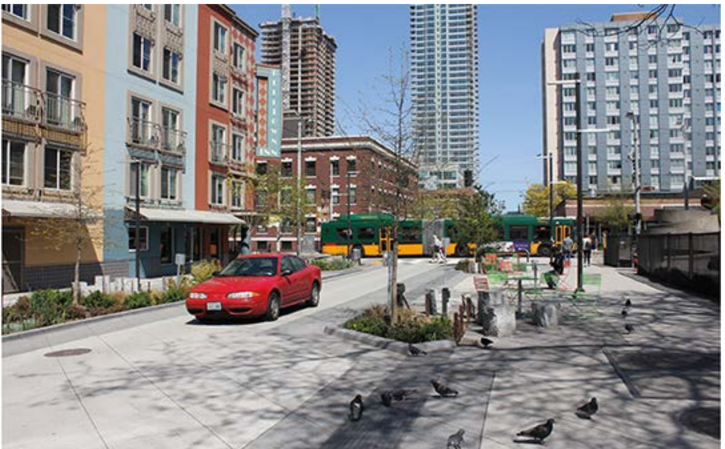
BELOW: Bell Street in the Belltown neighborhood of Seattle, WA was reconstructed as a shared street in 2014. The street is flush with the sidewalks. The only raised areas are landscaped planters.
