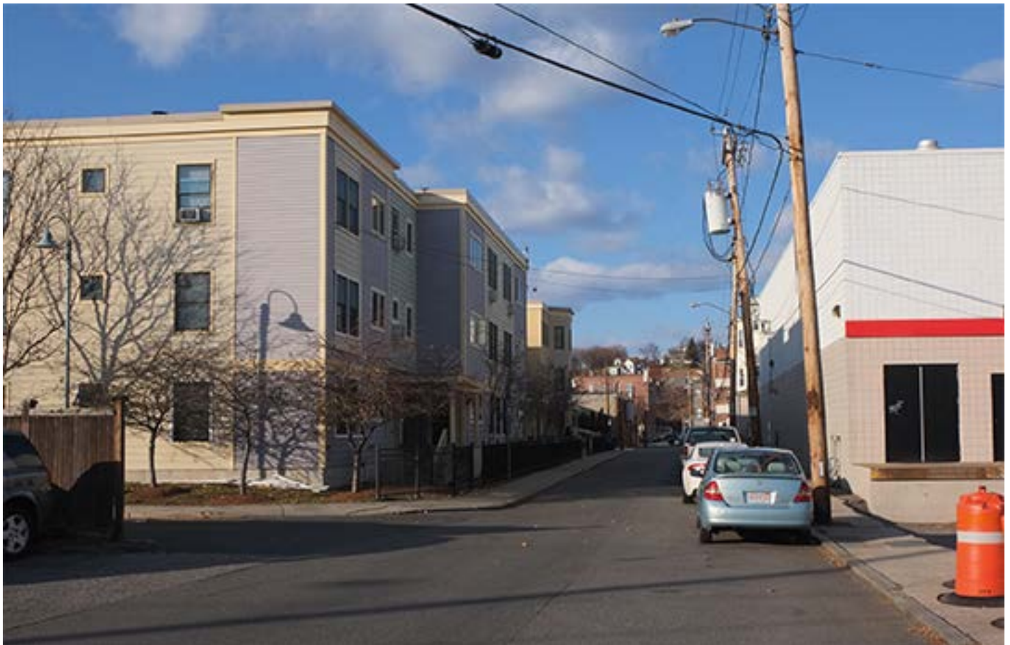
BELOW: The existing context of Merriam Street. Apartment buildings face the back of Advanced Auto Parts and Target's loading dock.
