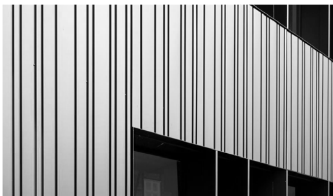
ARTICULATED METAL PANELS WALL TYPE- 02
