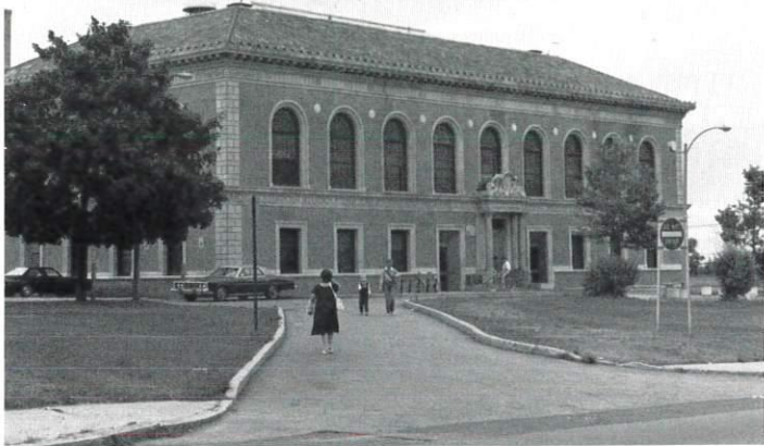
Somerville Public Library, 1914. Edward Lippincott Tilton, architect. Edward L. Tilton (1861-1933) was a noted designer of modern public libraries and was commissioned for the 1914 Somerville Public Library. Born in New York, Tilton studied at the Paris Ecole des Beaux Arts and worked for the New York firm of McKim, Mead and White, prior to establishing his own practice. In addition to his many library commissions, his partnership with William A. Boring (Boring and Tilton) produced the Ellis Island Immigrant Station in 1900. The Somerville and Springfield, Massachusetts libraries are considered characteristic examples of his work.
