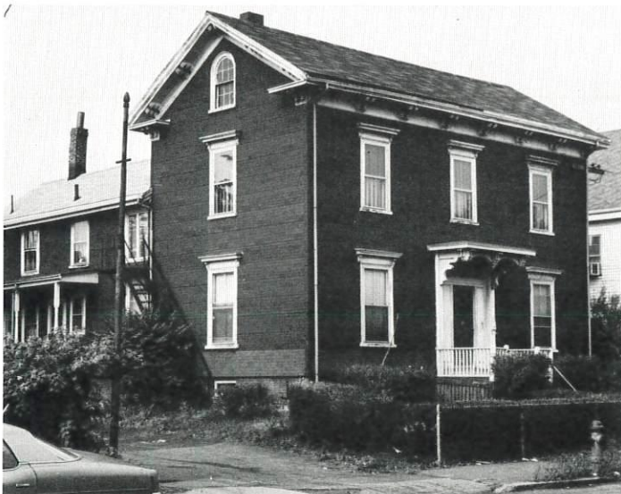
105 Prospect Avenue, ca. 1870. Ward II Italianate house has round-arched windows in the gable end.
