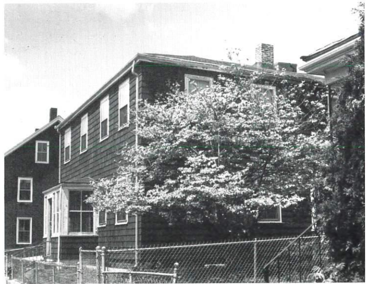
Osgood Dane House, 461 Somerville Avenue, ca. 1825. Quarry-owner Osgood Dane worked the granite ledge behind his residence (near Granite Street). The Dane House is the oldest house still standing on Somerville Avenue.
