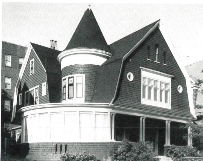
Eldridge Newton House, 8 Westwood Road, ca. 1897. One of the early houses of Westwood Road, and representative of the Shingle Style preferences of Westwood Road builders.
