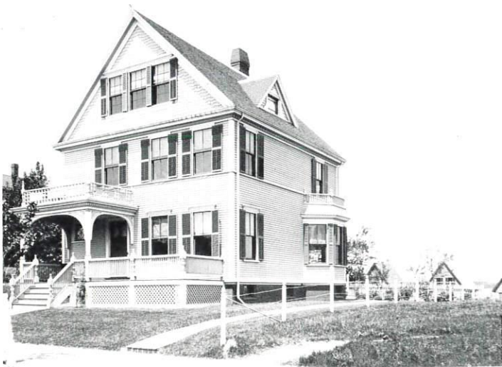
Charles X. Dalton House, 99 Highland Avenue, ca. 1890. Photograph ca. 1900. A shingled gable, turned porch posts, and clapboard siding are characteristic Queen Anne details. Dalton was a manufacturer of optical instruments.
