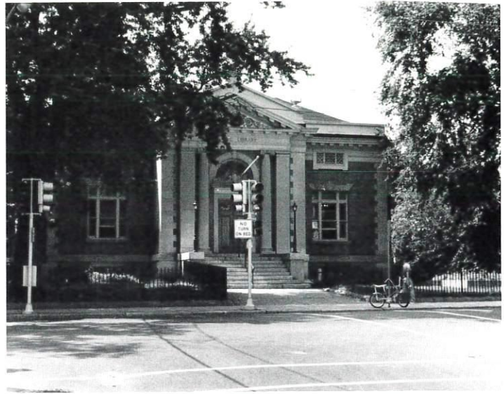
West Somerville Branch Library, 40 College Avenue, 1909. Renaissance Revival and Neo-classical motifs were favored by the designers of early twentieth century public and commercial buildings. Round-arched windows grouped in arcades and broad, overhanging roofs characterized the Renaissance Revival designs often chosen for firehouses and schools; classical motifs such as over-scaled columns carrying a classical pediment are evident on the Neo-classical West Somerville Branch Library. McLean and Wright of Boston were the architects.
