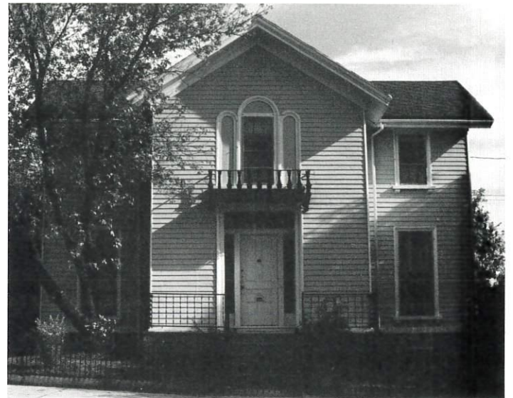
Charles Williams House, 108 Cross, ca. 1848. One of the best conserved early Italianate houses in Somerville. The Palladian window motif and glazed transom and sidelights of the projecting pavilion are features of the original design. Williams was a Boston hat dealer.
