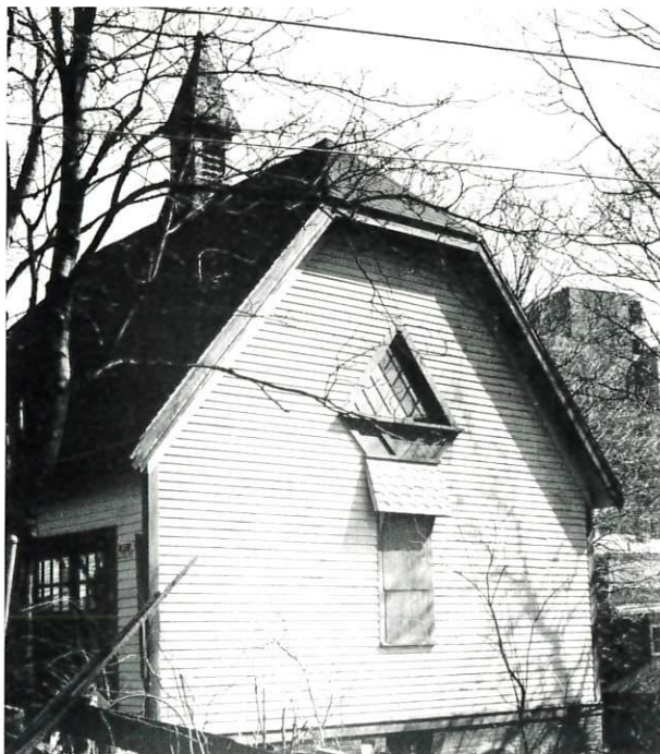
Carriage house, Columbus Avenue. A jerkin-head roof and multi-paned windows are distinctive features of this Queen Anne Style carriage house which dates from the 1890s.
