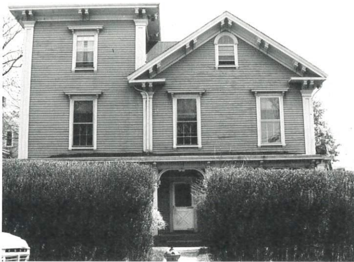
Alexander Foster House, 45 Laurel Street, ca. 1860. The Foster House is an excellent example of the Italianate Style; of note is the square bracketed tower and an ornate porch.
