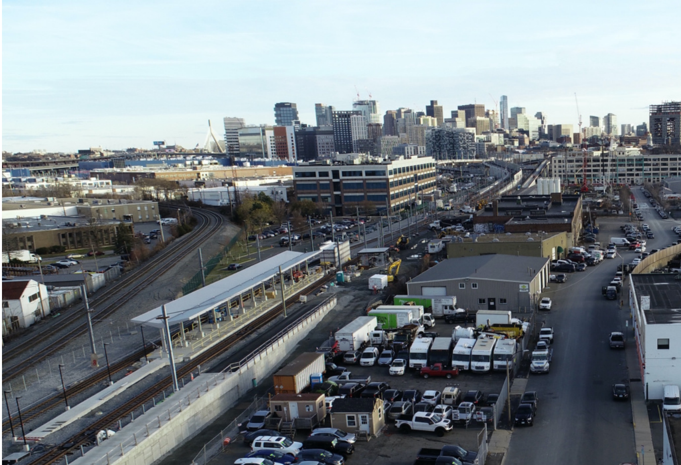
New MBTA Green Line station under construction
