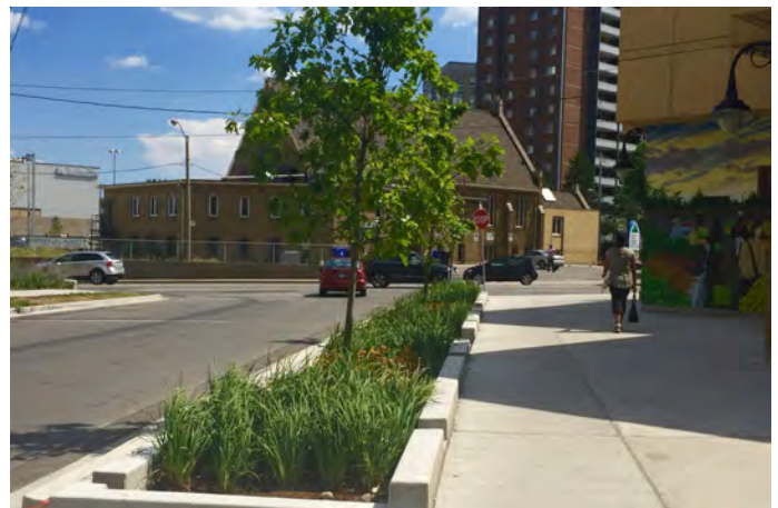
Tree wells can be used as a green infrastructure device to capture stormwater
