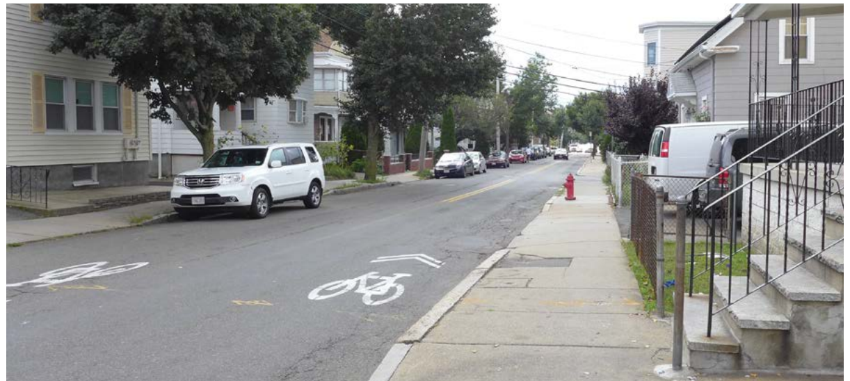
Figure 3-12. Streetscape at Lowell St: The narrow street accommodates one lane of parking and two shared lanes for cars and bikes.
