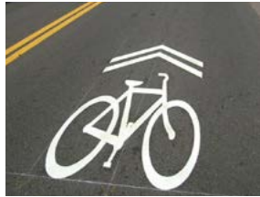
Figure 3-23. Shared bike lanes, or bike “sharrows,” represent the design with the lowest level of comfort for cyclists. Source: Brent Adams and Associates, 2012.
