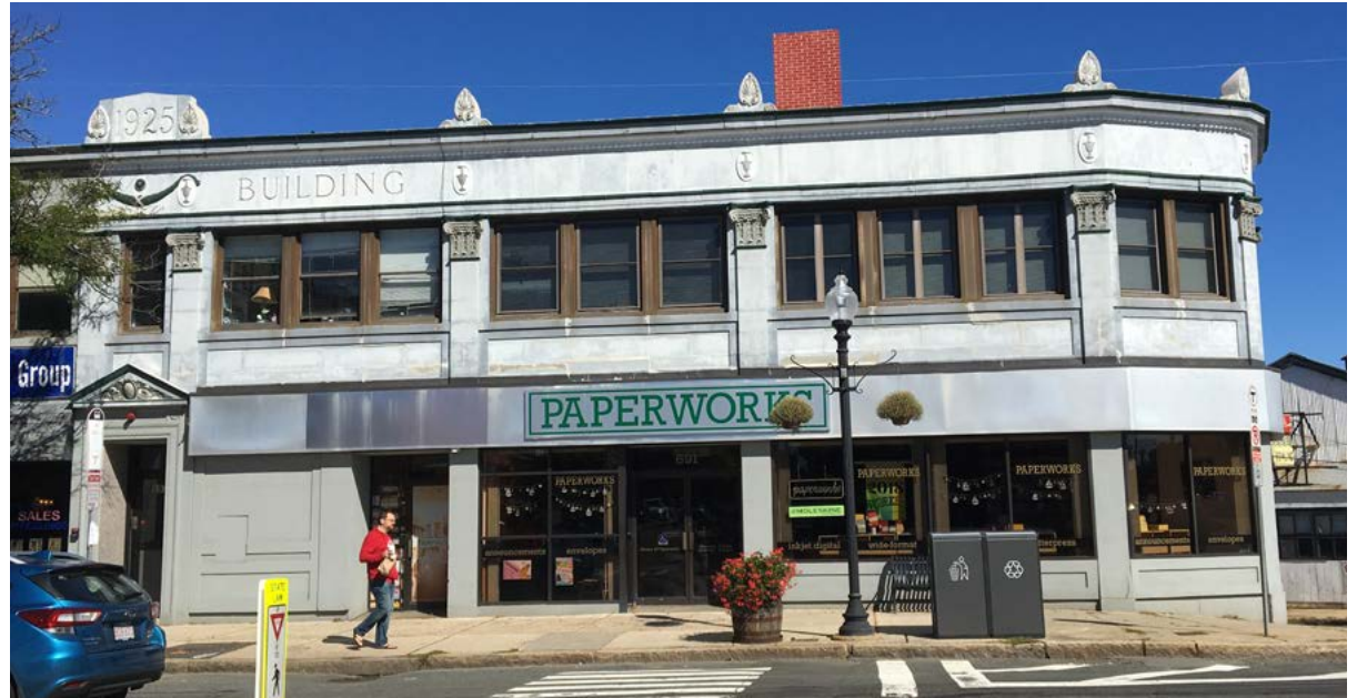
Figure 4-14. Existing conditions at the site of the proposed development at 691-703 Broadway
