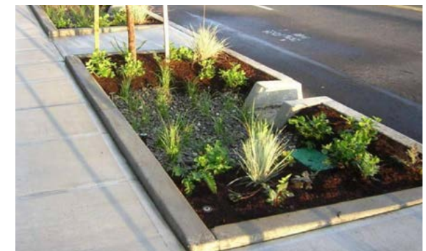
Figure 3-8. Example of a sidewalk planter to manage street runoff. (Source: Philadelphia Stormwater Guidance Manual. 2014.)
