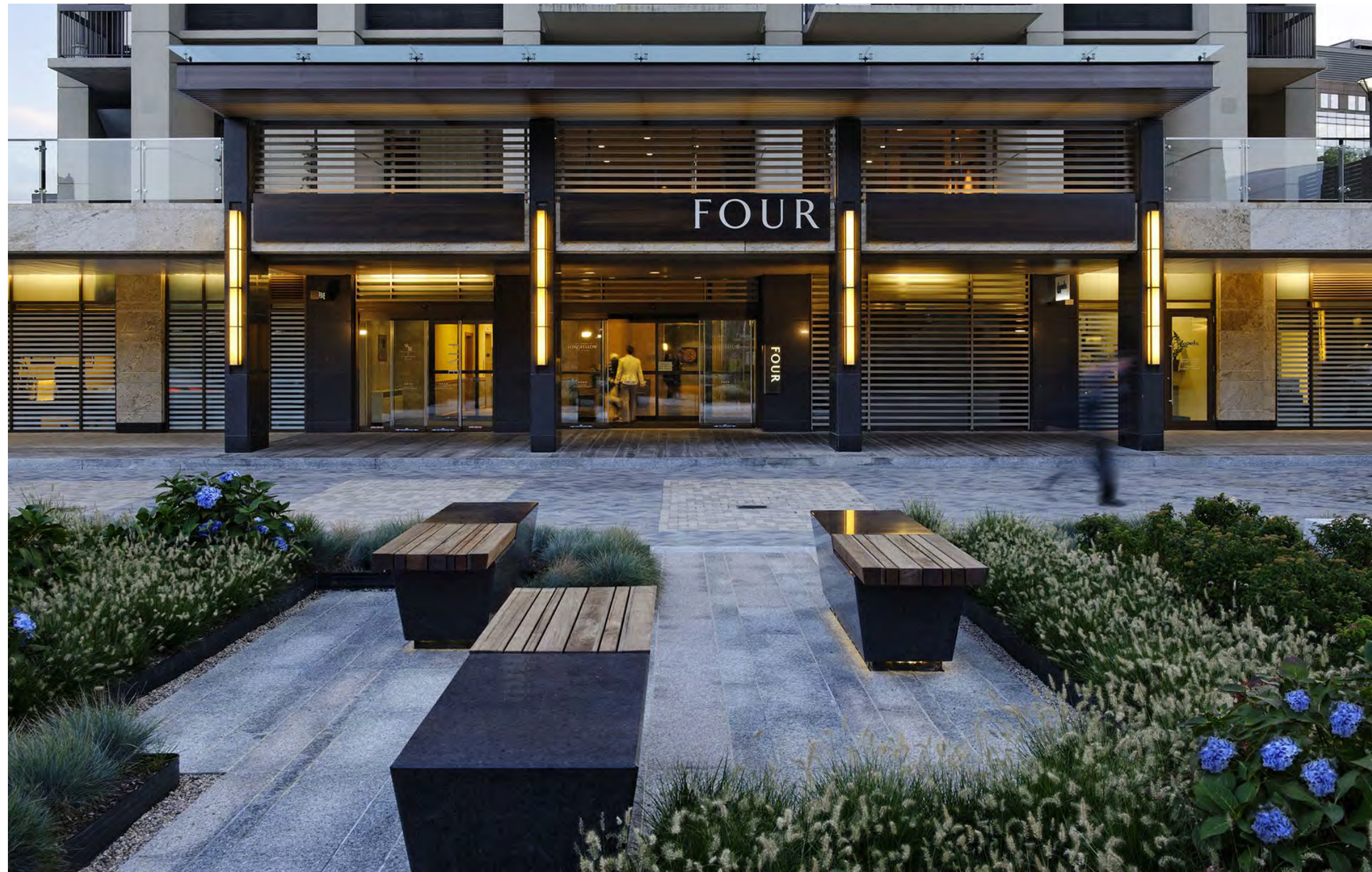
Linear seat walls with wood tops
