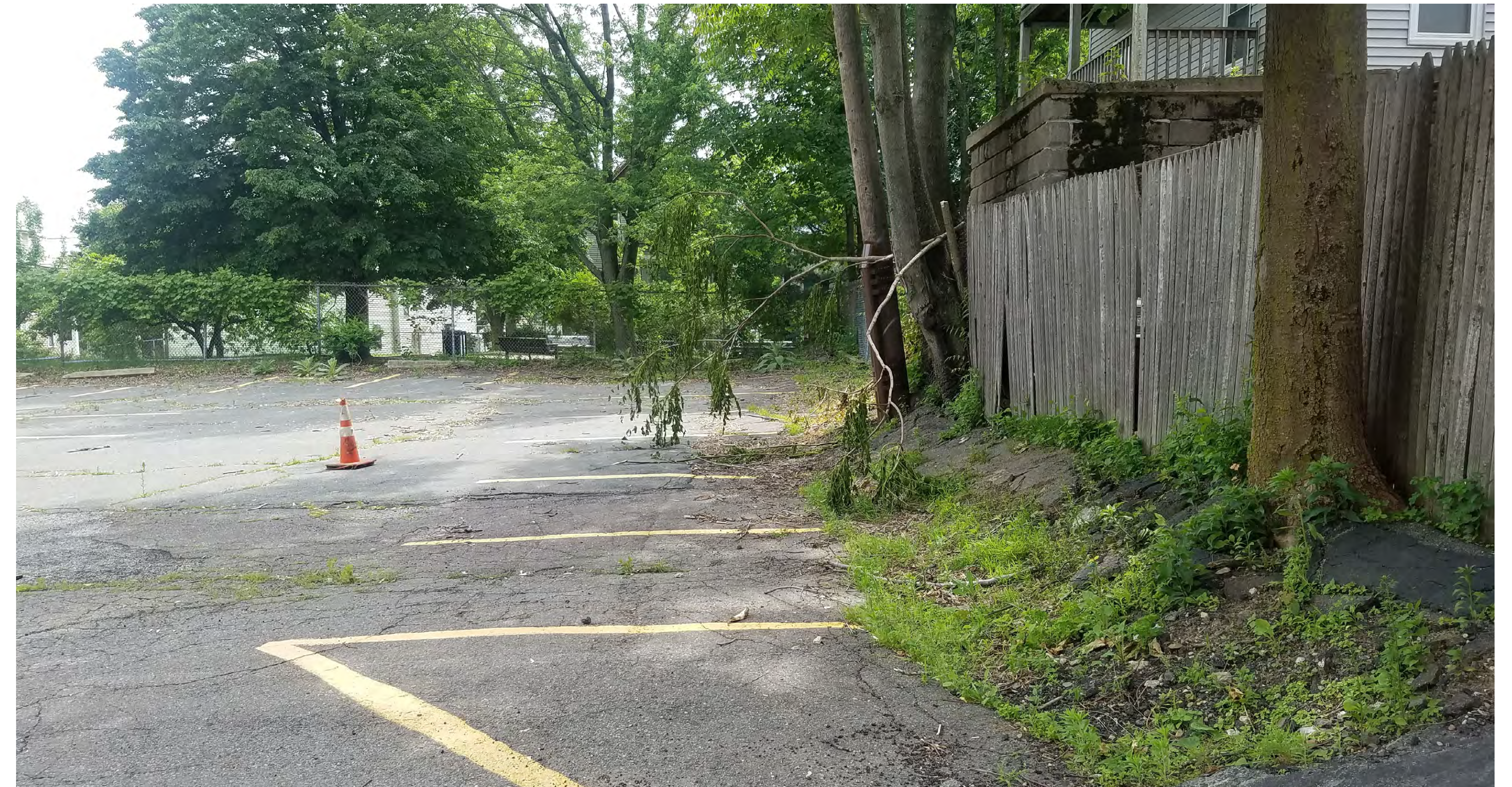
Deteriorated asphalt surfacing and damaged wood fencing
