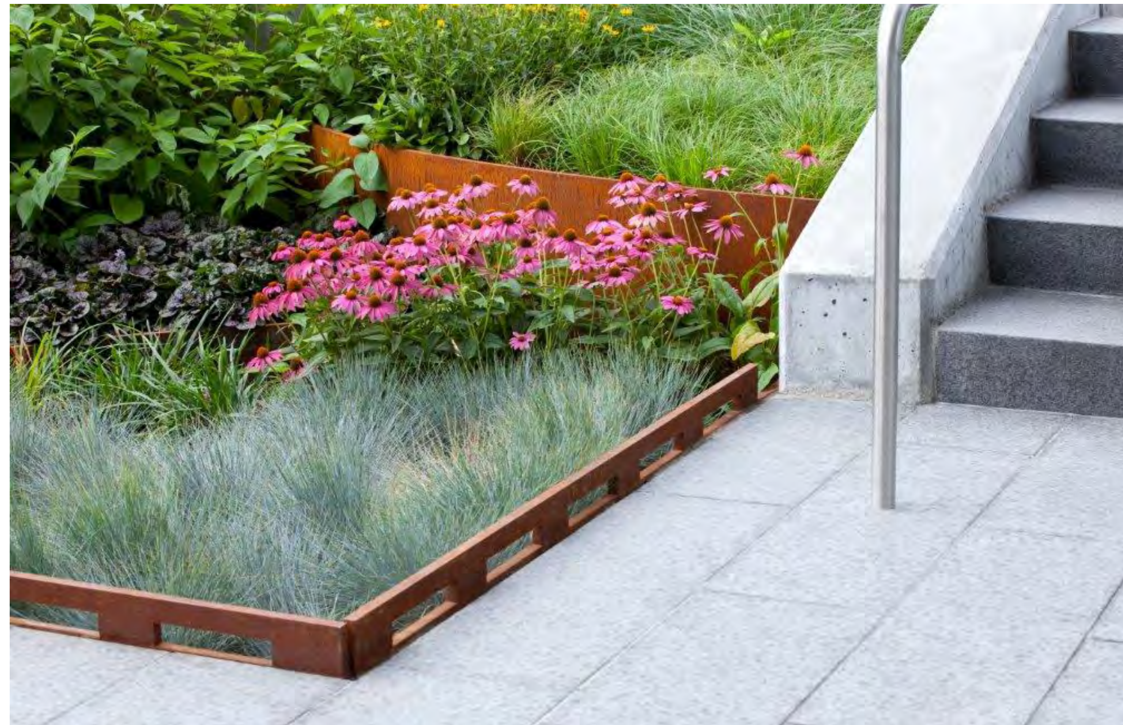
Corten steel planter edge with openings for stormwater (at pocket park planting)
